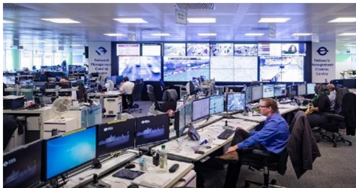
A view of TfL's control room. Key route traffic lights' phasing can be adjusted to help traffic flow in real time.
