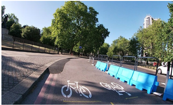
Former key arterial route Park Lane looking north. Three traffic lanes now two, speed limit reduced from 40, to 30, to a 20mph crawl TfL fines a constant threat against otherwise innocent motorists
