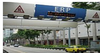
Singapore sling. A pay-per-mile road charging monitoring gantry
