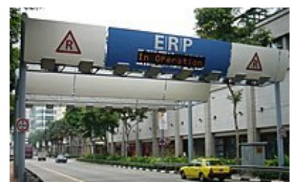
Electronic Road Pricing gantry Singapore
